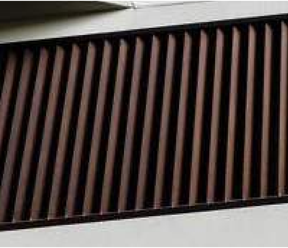
LV2 LOUVRES TYPE 2 VERTICAL ALUMINIUM BLADES
