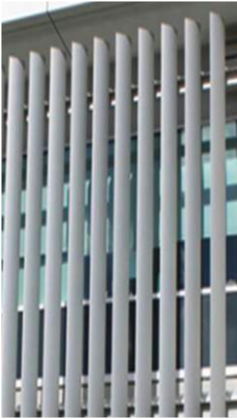
LV1 LOUVRES TYPE 1 VERTICAL ALUMINIUM BLADES
