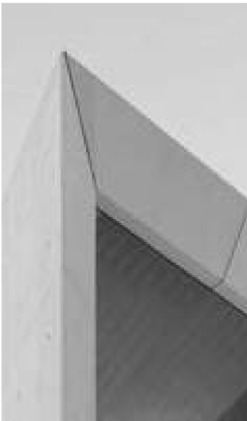
LC1 LIGHTWEIGHT CLADDING TYPE 1 LIGHT TONED VERTICAL CLADDING & SUNSHADES ALUMINIUM OR SIMILAR
